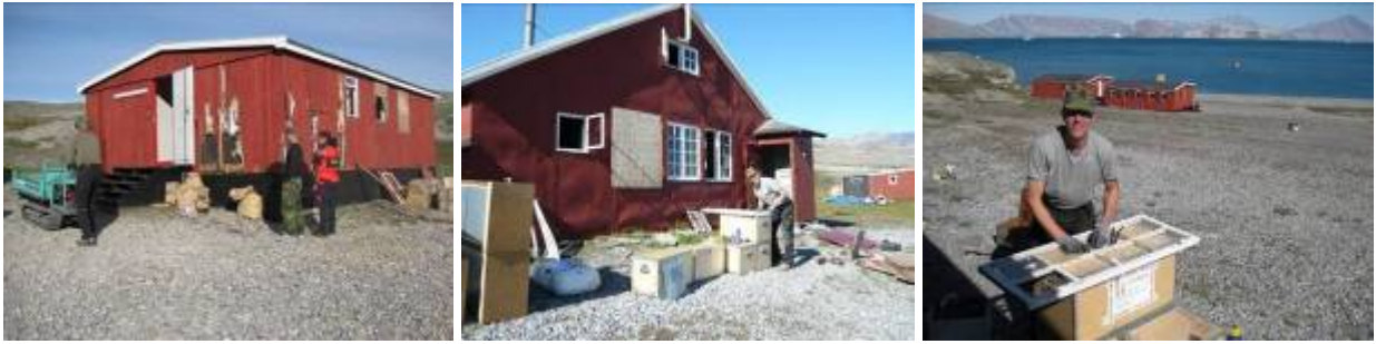
Inspecting and repairing damages caused by polar bear. Right: Birger Bjerregaard.
