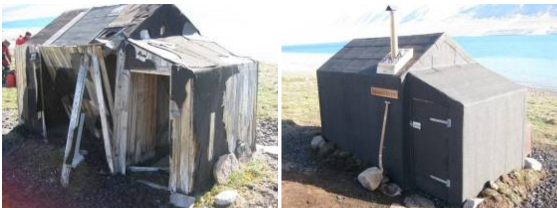
Brøggers hytte in Duséns Fjord before and after renovation.
